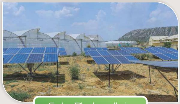
Solar Photovoltaic Water Pumping System
